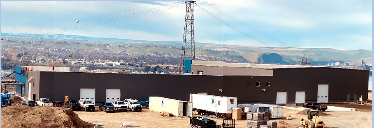
Northwest Fourslide Facility, March 2024
